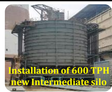
Installation of 600 TPH new Intermediate silo Ash Augmentation project in Fly ash system.
