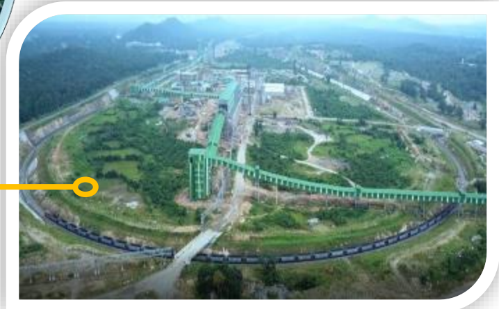
48 Km Long Dedicated MGR Railway Line from OPGC to Manoharpur for Coal Transport
